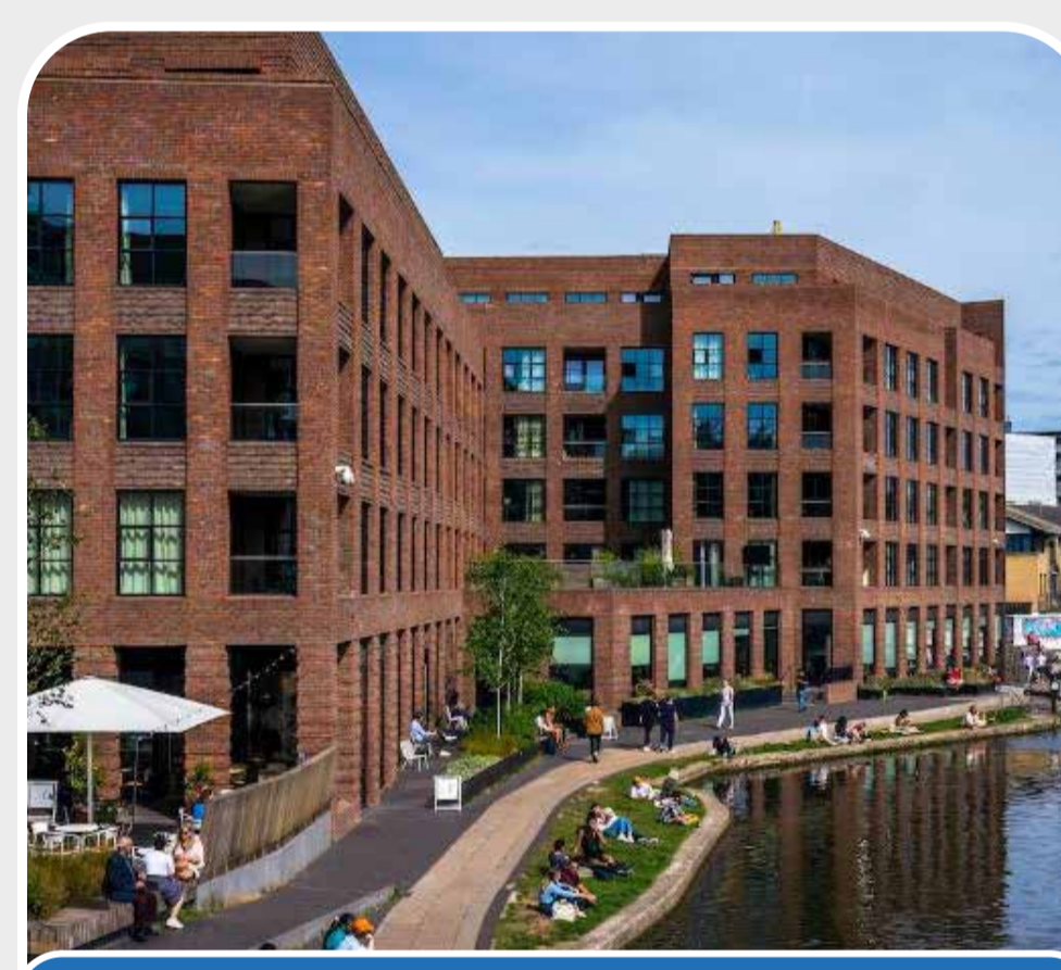
Hawley Wharf, Camden, AHMM
